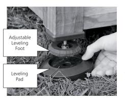
**3** Determine if shed is installed in a level position using a level on the floor of the shed. If further leveling is needed, use additional leveling pads to adjust the height of each corner. For smaller adjustments, turn the leveling feet in or out. If more than an inch of thread is showing above the foot, use and additional leveling pad instead. **Do not use more than four leveling pads in one corner.**
